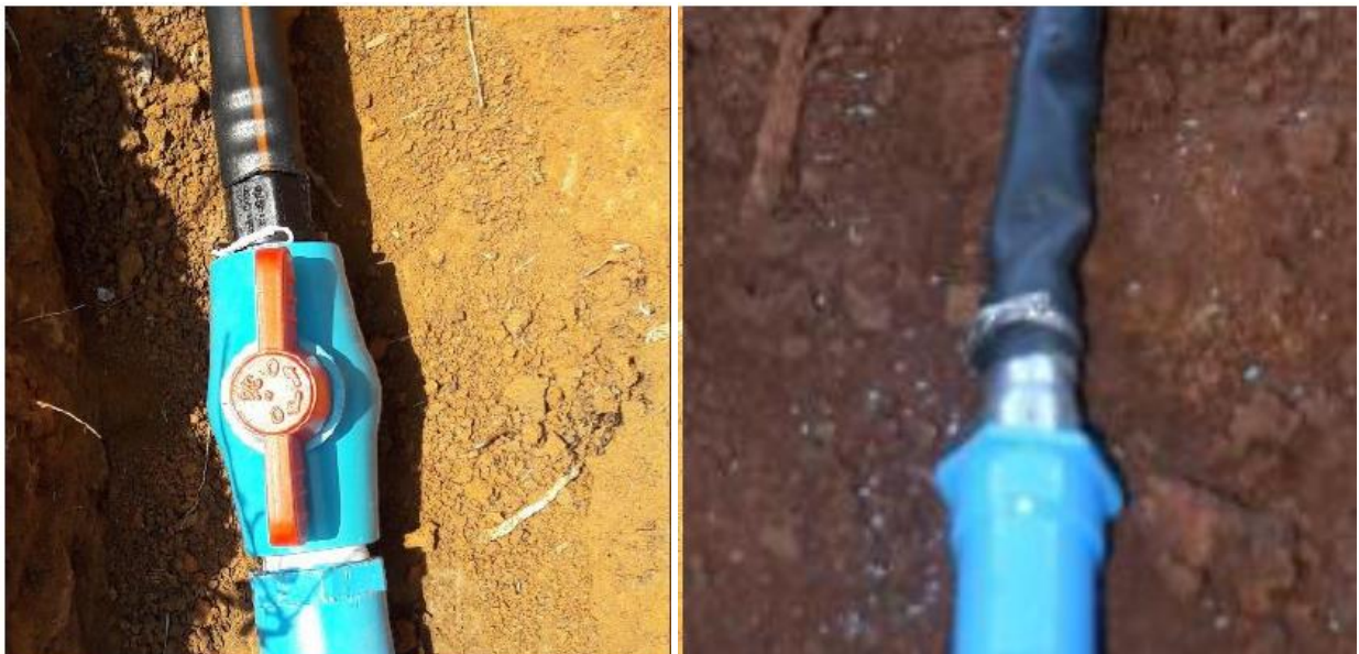
Figure 27: Left: A good PE pipe is attached to a connector, tightly fitting the profile. Right: A low quality PE pipe is fixed to a connector by use of a wire.
