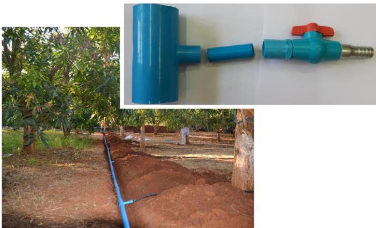
Figure 24: Downhill installation of the main line and direct connection of laterals
