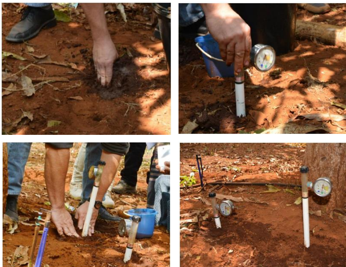
Figure 31: Installation of a tensiometer
