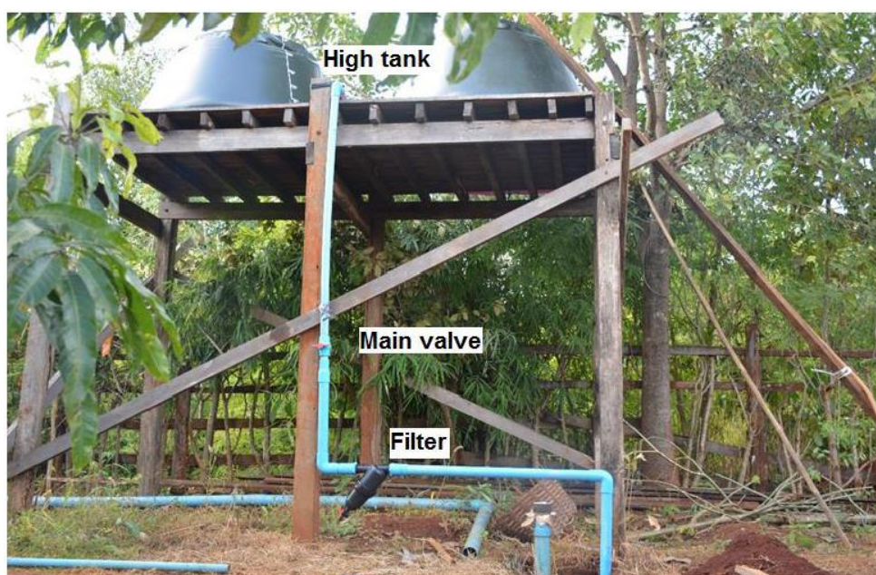
Figure 23: Elevated tank, main valve and filter at the inlet of the main line of the gravity-fed drip-irrigation system.
