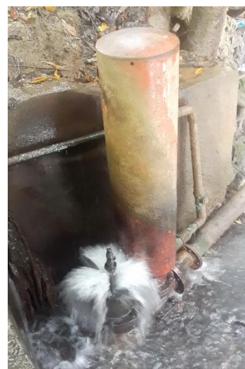
Figure 5: Functioning principle of a hydraulic ram (left); Hydraulic ram for water lifting in Hopone, Southern Shan State, Myanmar (right)
